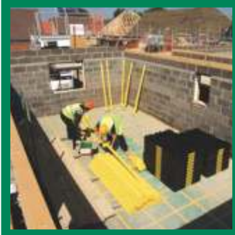
Components can be visibly checked before erection commences
